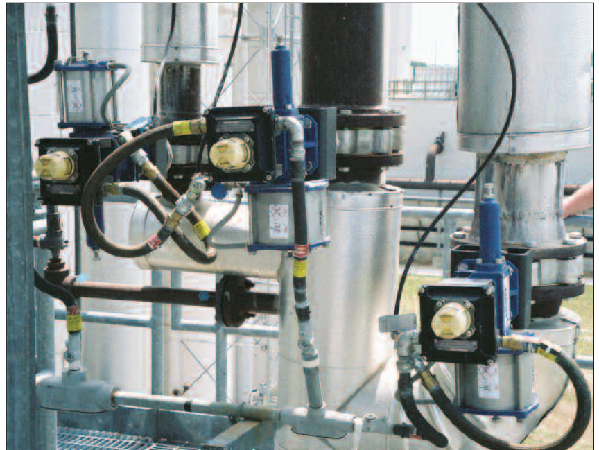
Pictured above are Vanessa Fig. QTLs with Morin Series B Pneumatic Actuators, and Westlock Limit Switches
